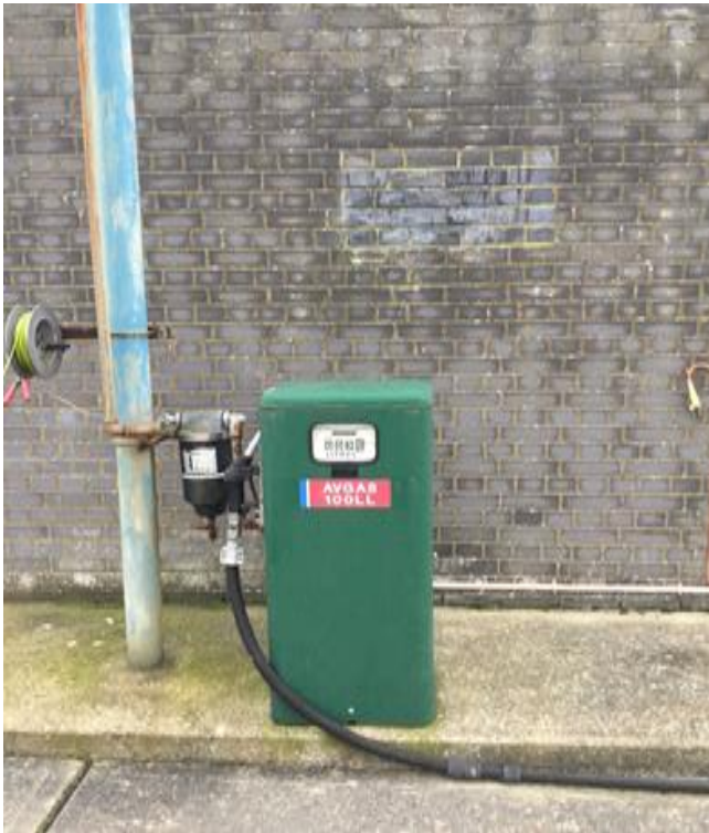
Picture 6 Avgas 100LL pump at former aviation training centre.
